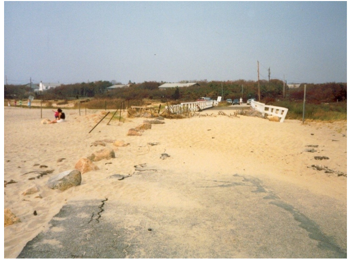
The Menauhant Road bridge after Hurricane Bob eroded the beach and blew sand onto the road. (1991)
